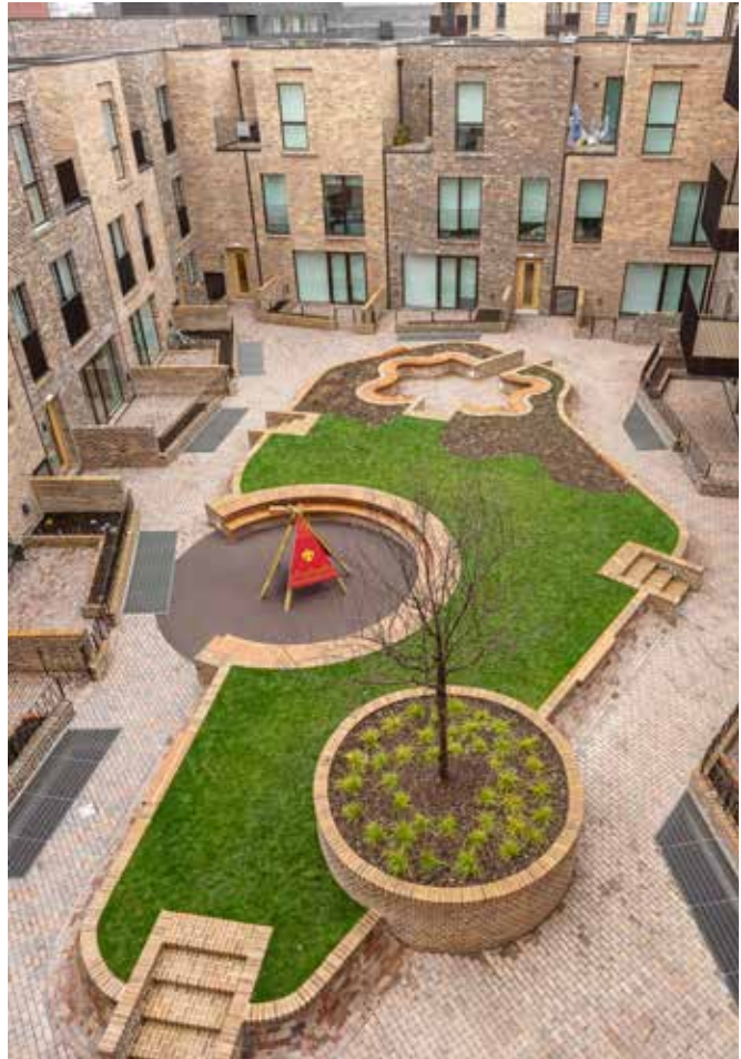
Terraces front onto communal amenity space.
