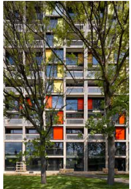
Park Hill Phase 1, Sheffield, UK. Sheffield council. Refurbishment Hawkins\Brown and Studio Egret West.
