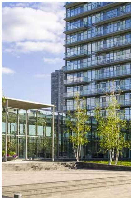
NXT & NXT2 at Windermere By the Lake, Toronto, Canada. Architect Alliance.
