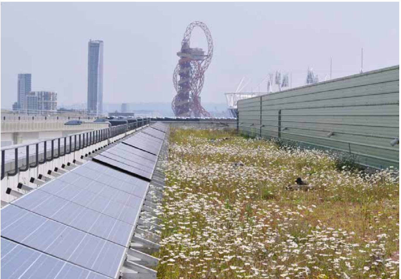
Rooftops incorporate solar energy and biodiversity.
