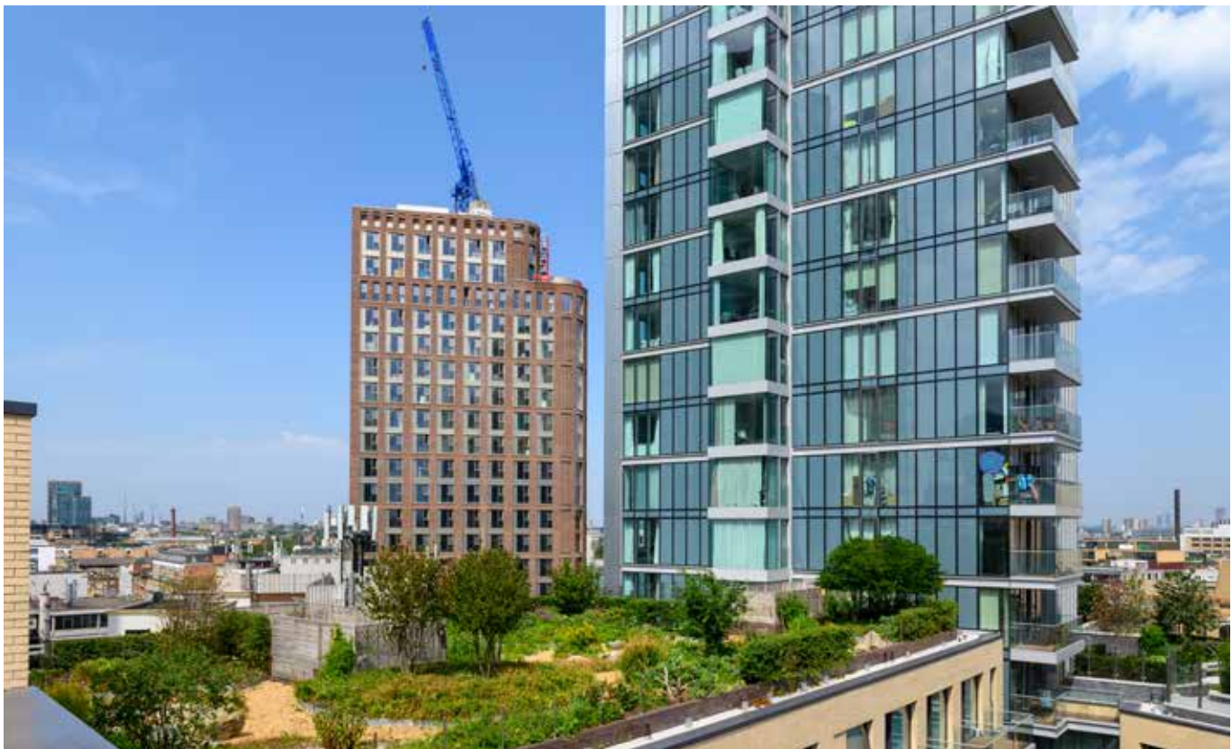
Rooftop with extensive biodiverse landscaping
