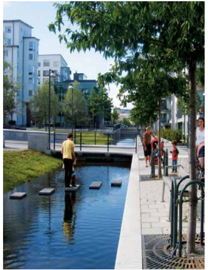
SUDs detention basin incorporated into public realm.
