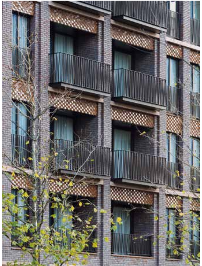
Semi-recessed balconies with distinctive balustrades.
