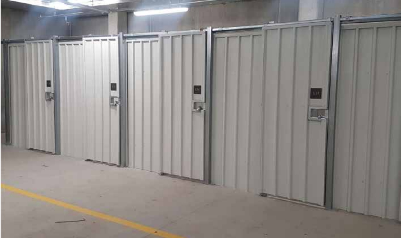
Secure basement storage lockers.
