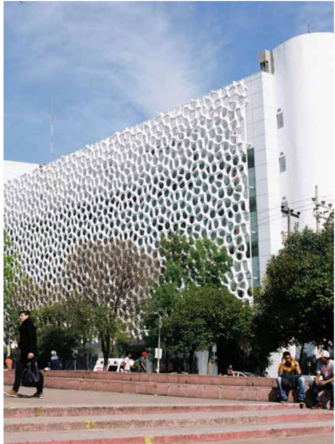
External cladding has anti-microbial and de-polluting properties to filter the surrounding air.
